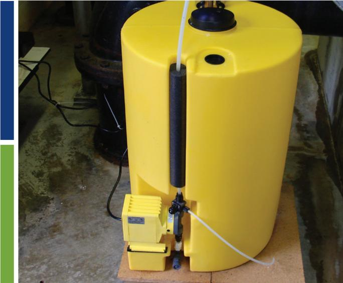
capacity and are partnered with a pump capable of delivering 1-2 gallons per hour. Dilute Strike® liquids in sufficient water to match the viscosity of water. This increases the accuracy of the pumping mechanisms as most equipment is graduated and calibrated using water.
